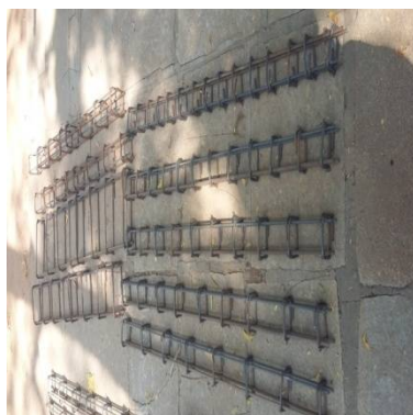
Reinforcement Details
